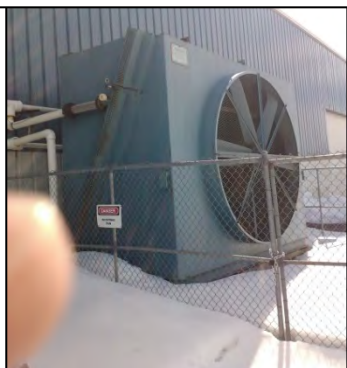
Exterior arena fan for natural cooling
