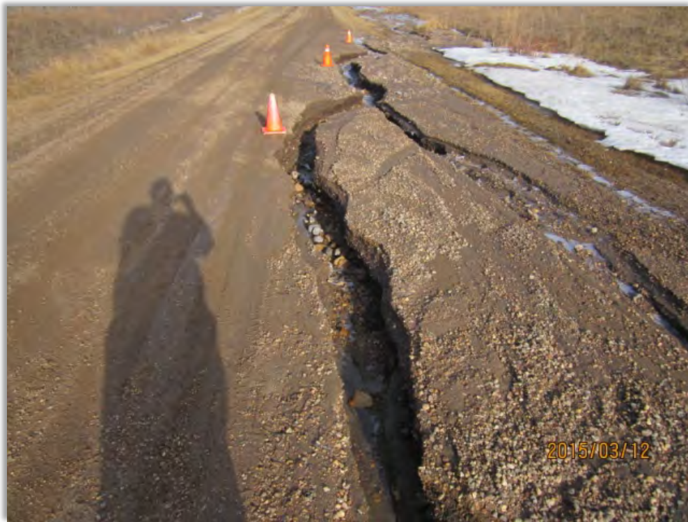
East side of access road
