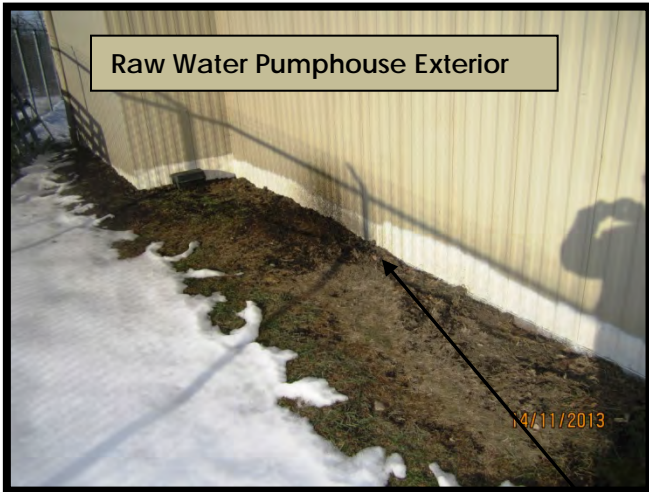
Raw Water Pumphouse Corrosion
