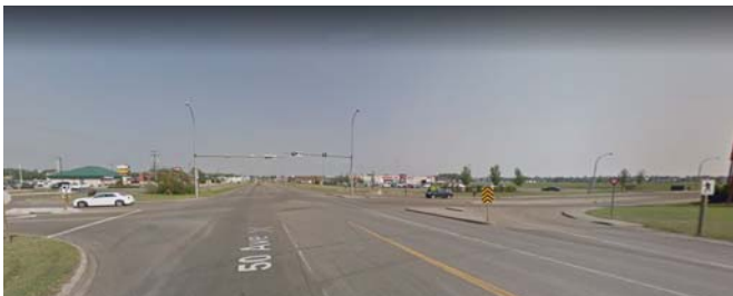
Intersection of Highway 12 and 67th Street in the Town of Stettler
