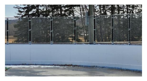
Chain link is installed in sub sections between stanchion points vs linear section chain link allowing for easy future repairs to top cap and the highest use chain link sections.
